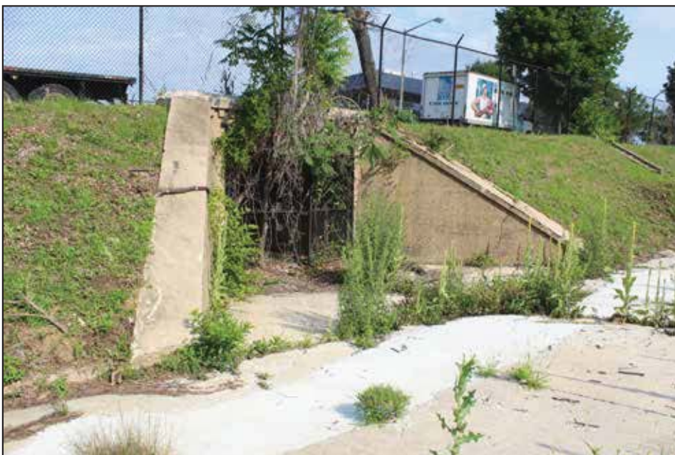
First Street Tunnel, looking northwest. 2015.
