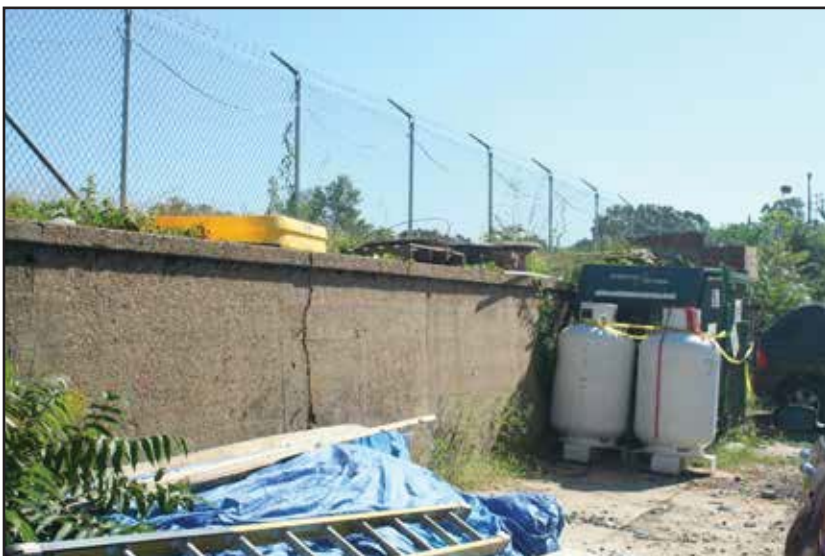
North Wall at Service Court 3. 2015.
