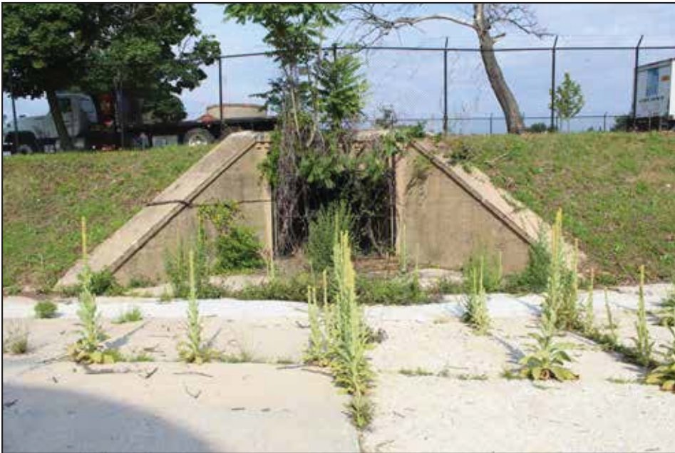
First Street Tunnel, looking west. 2015.
