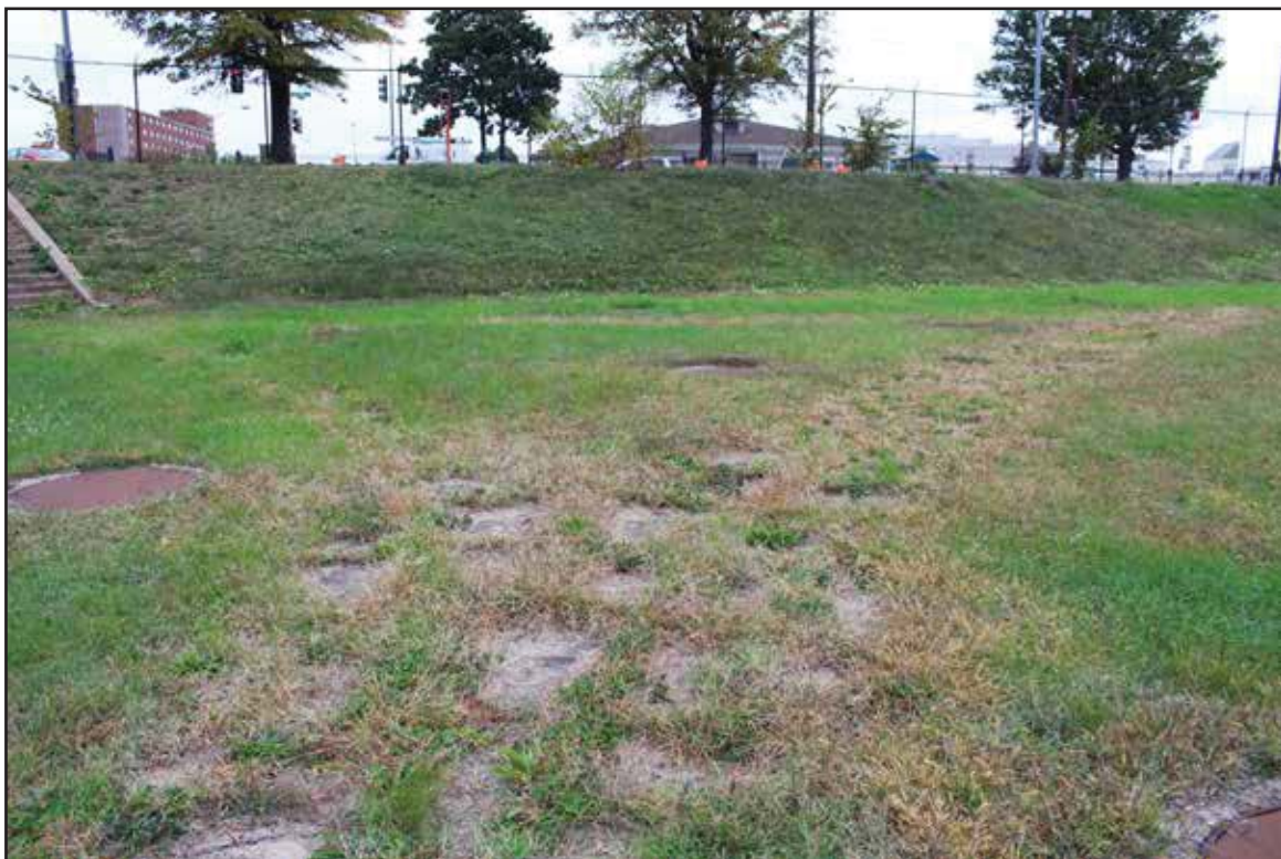
Remnants of pedestrian path at NW corner of site. 2015.
