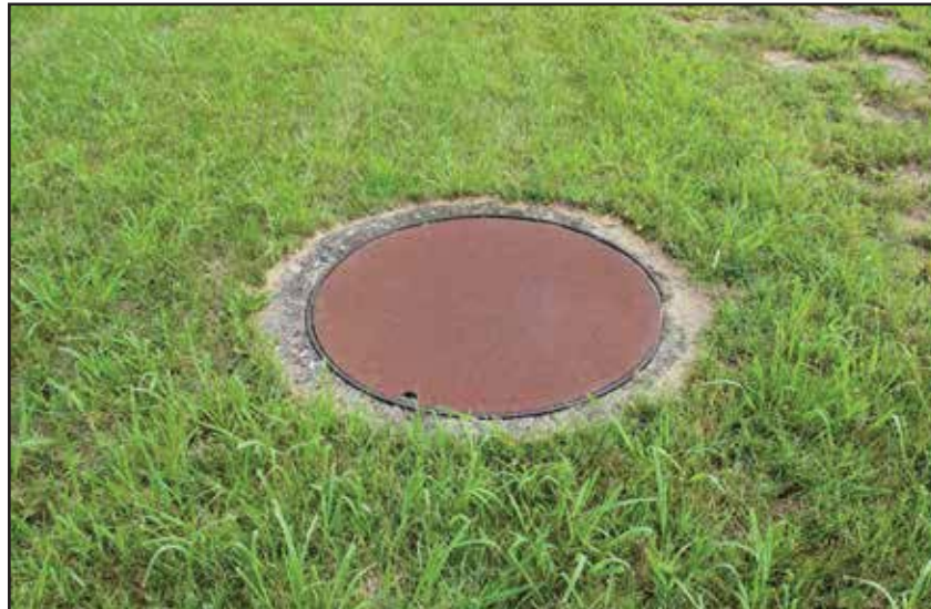
Intact manhole cover. 2015.
