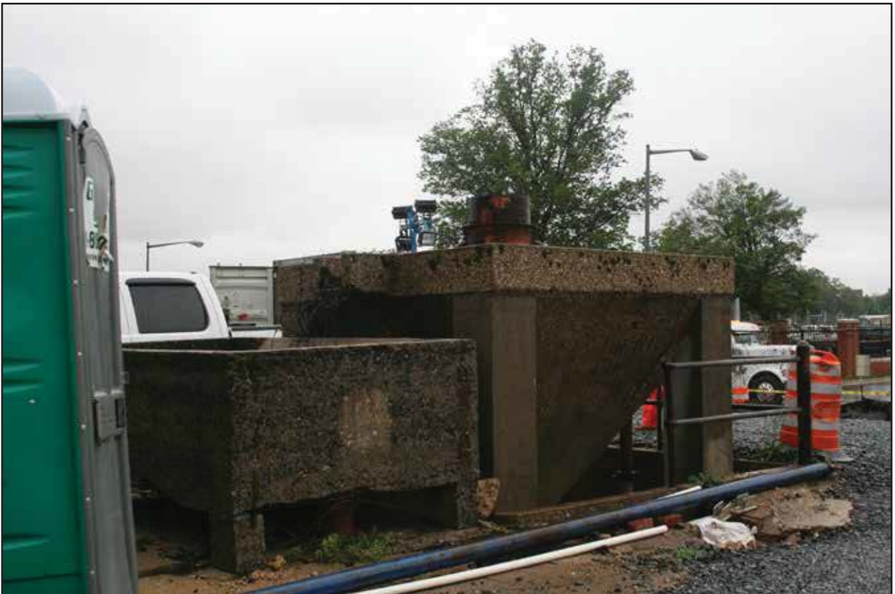
Sand washer 14 in Service Court 2, looking southwest. 2015.
