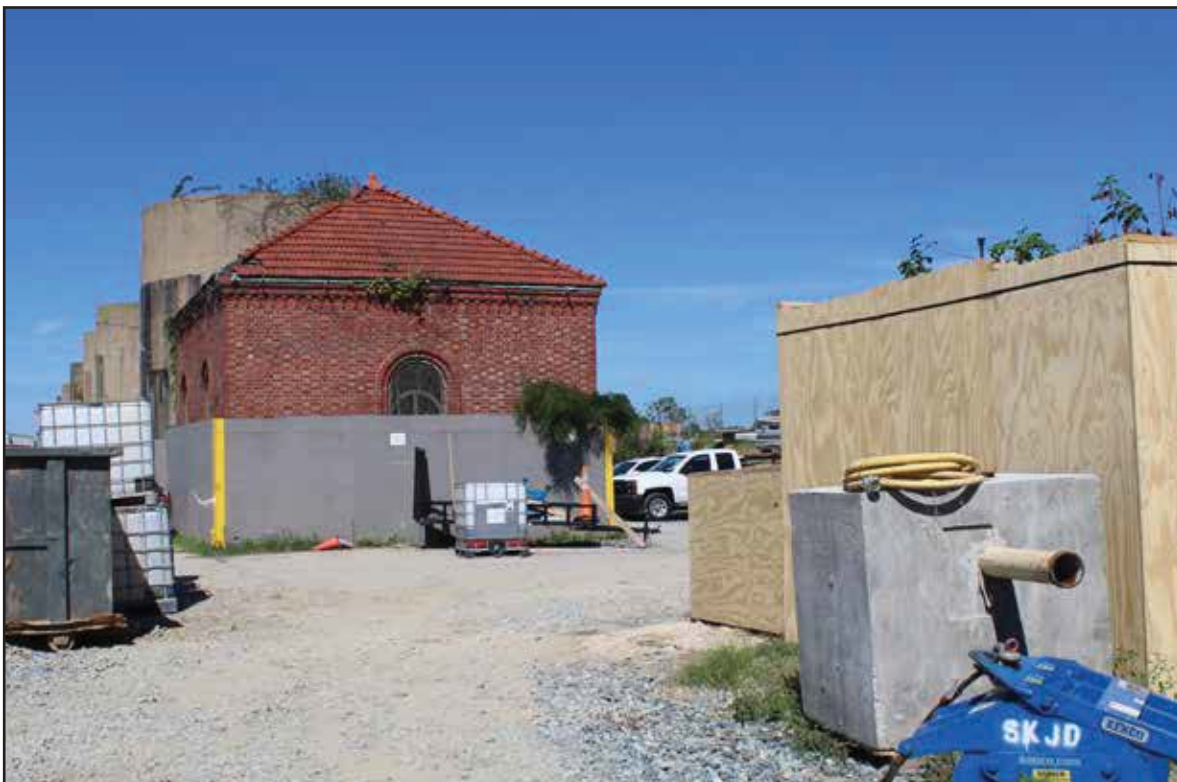
Service Court 3, looking west. 2015.
