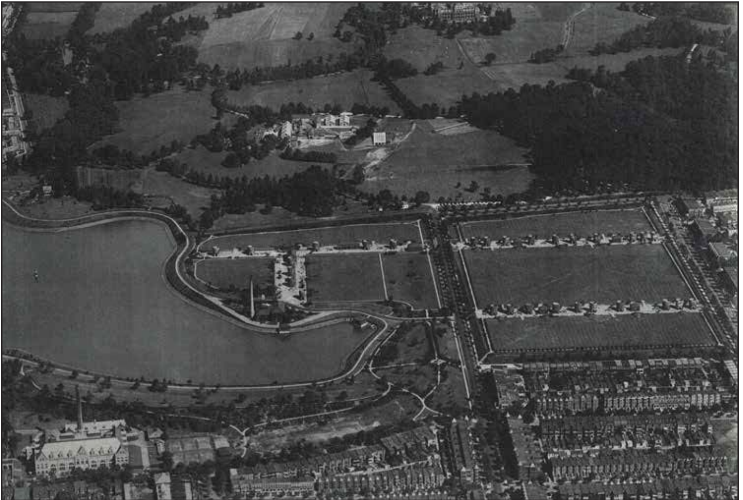
Figure 9 Aerial of McMillan Reservoir and Filtration Plant, 1921. National Archives and Records Administration.
