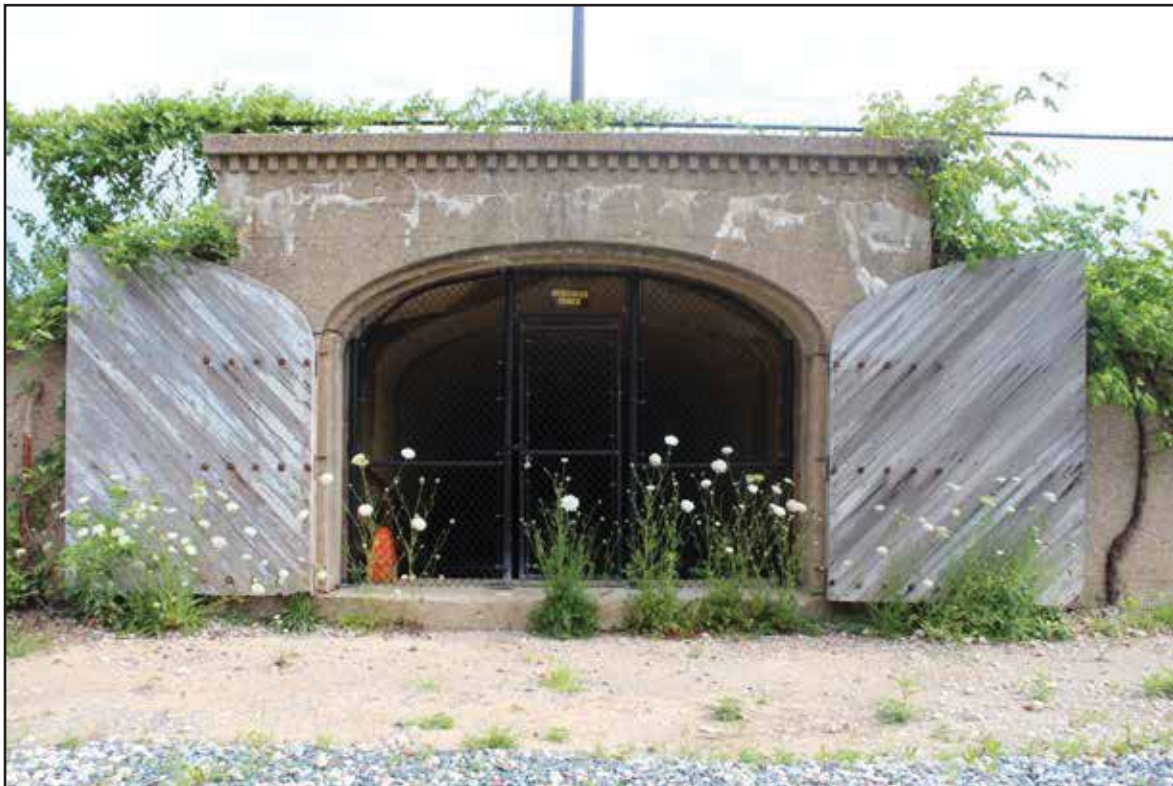
Filter Bed Portal 14. 2015.
