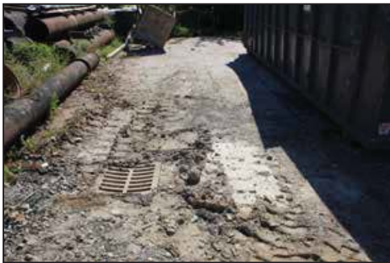
Detail of paving at Service Court 3, looking east from Filter Bed 24. 2015.
