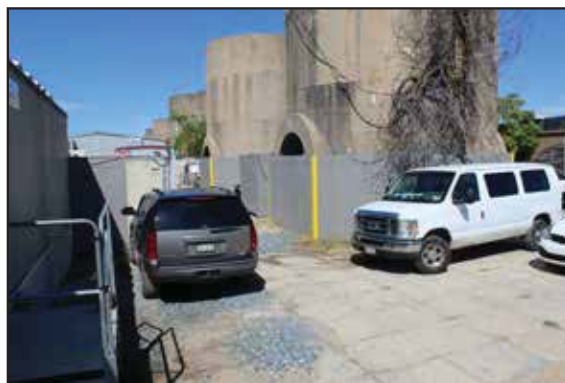
Detail of paving at Service Court 3, looking west from Ramp 14. 2015.
