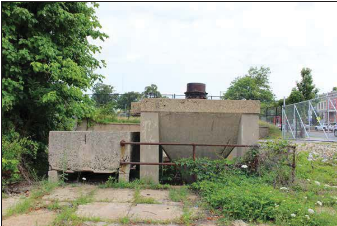
Sand washer 13 and discharge bin in Service Court 2, looking north. 2015.
