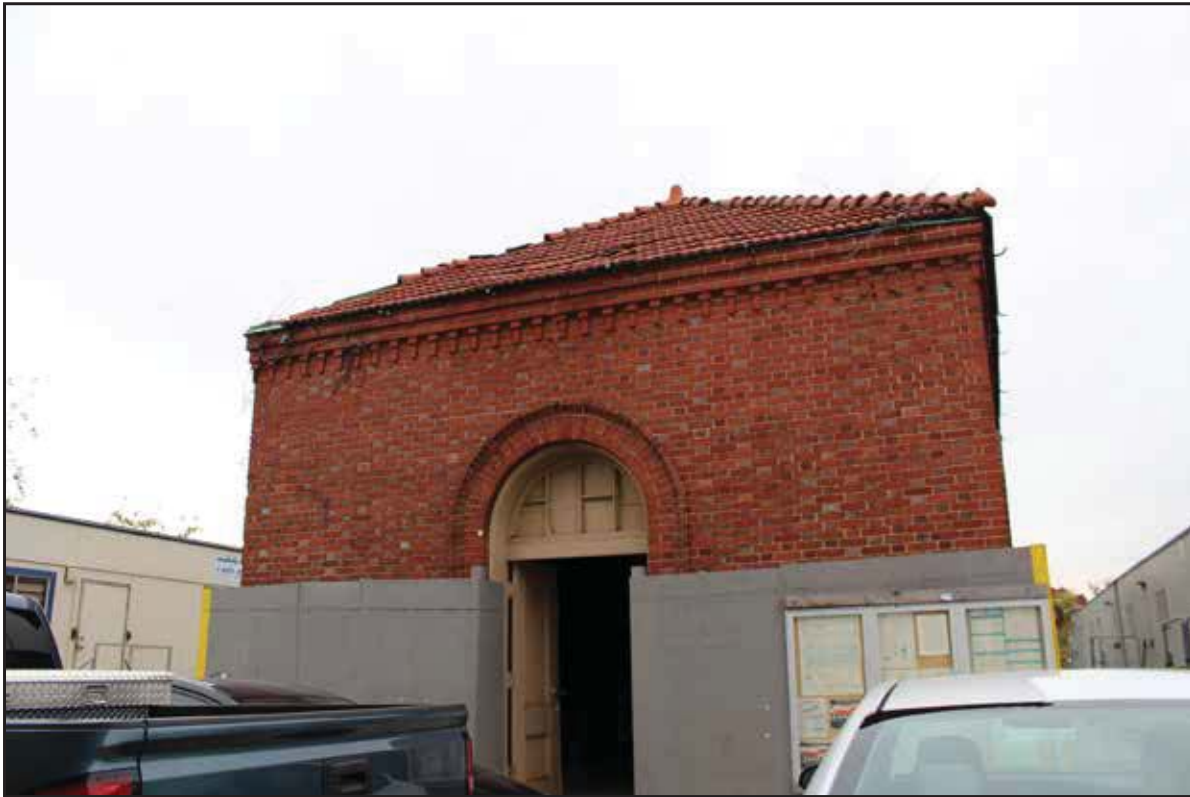
Regulator House 6, looking east. 2015.
