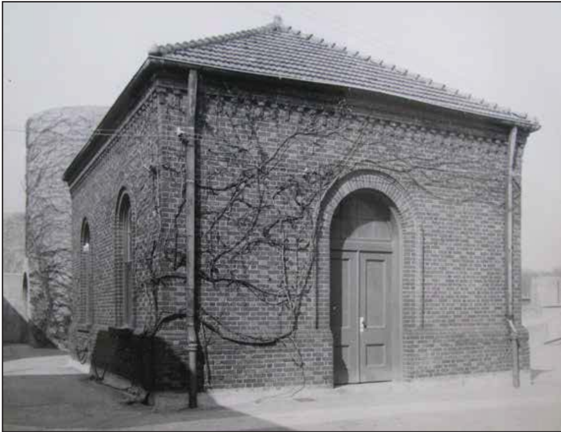
Regulator House 5, looking southeast. Circa 1944. Courtesy of the Washington Aqueduct Archives.
