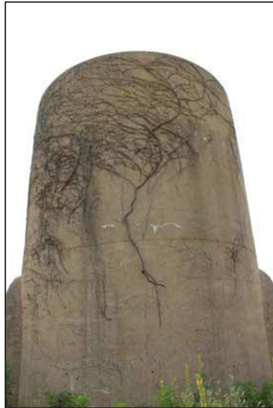
Sand bin 11, looking east. 2015.
