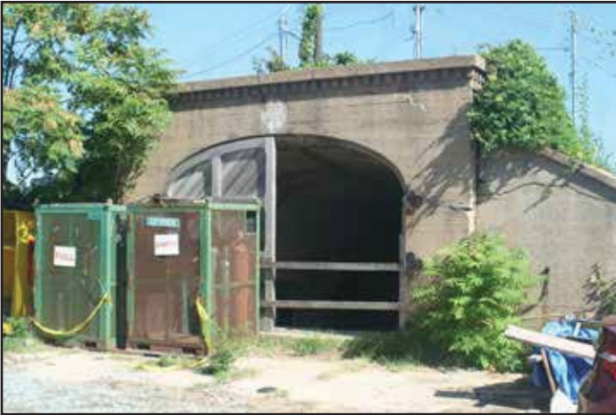
Filter Bed Portal 22. 2015.
