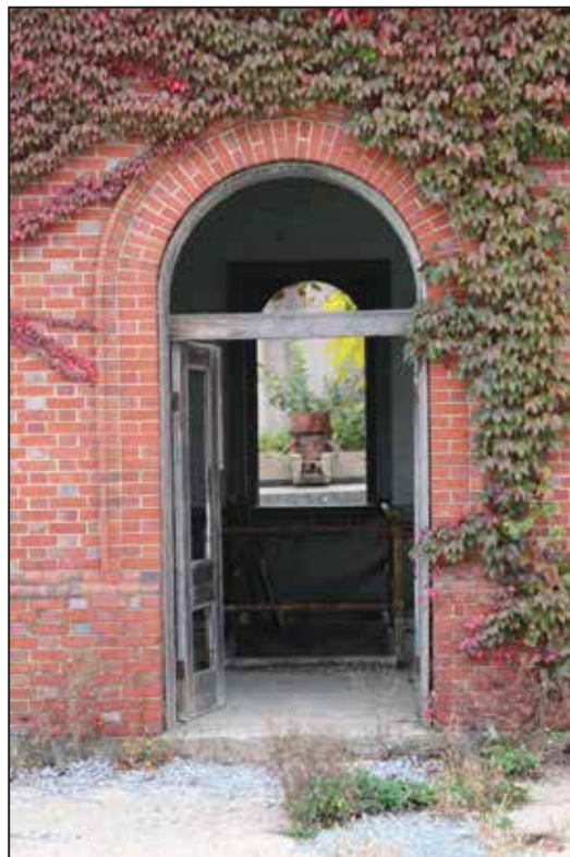
Regulator House 5, looking east. 2015.
