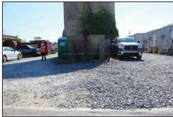
Detail of paving at Service Court 3, looking east from First Street. 2015.
