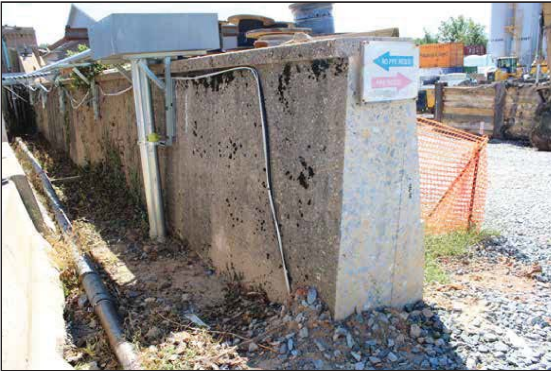
South Wall at Service Court 3, near Filter Bed. 2015.
