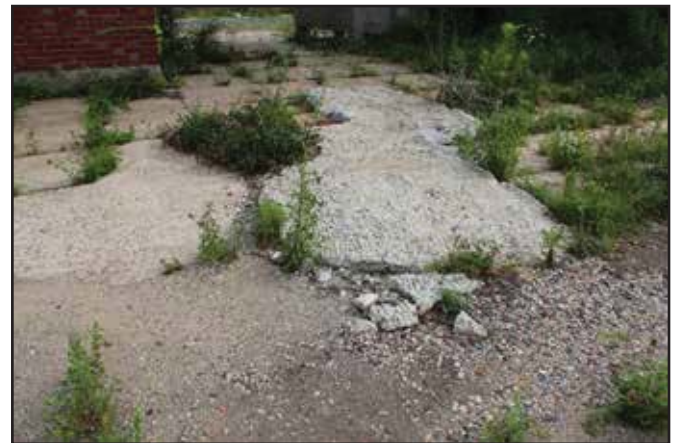
Detail of paving at Service Court 2, looking north from Regulator House 5. 2015.
