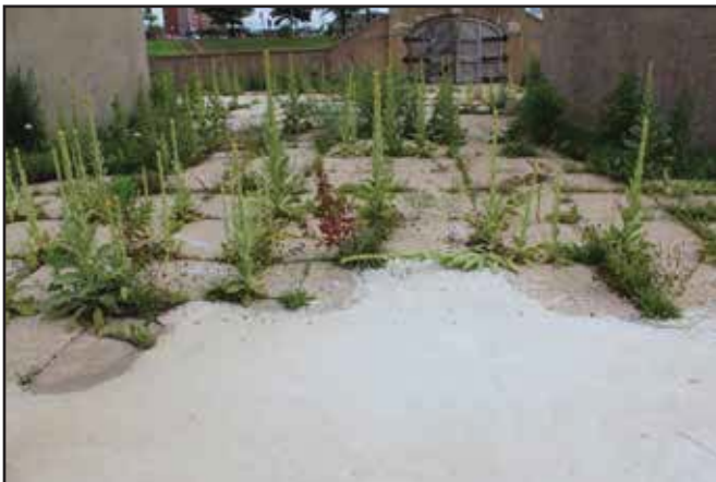
Detail of paving at Service Court 2, looking southeast from First Street. 2015.
