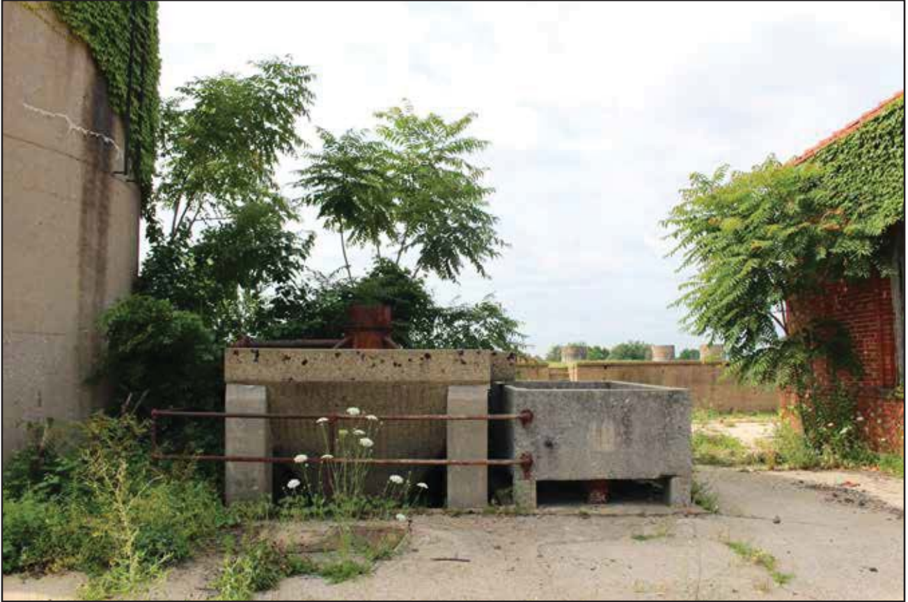
Sand washer 12 in Service Court 2, looking south. 2015.
