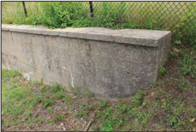
North wall at Service Court 2, near North Capitol Street. 2015.
