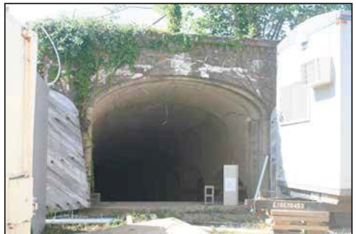
Filter Bed Portal 27. 2015.
