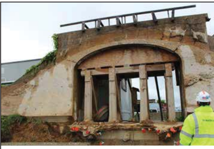
Temporary supports at Filter Bed Portal 25. 2015.
