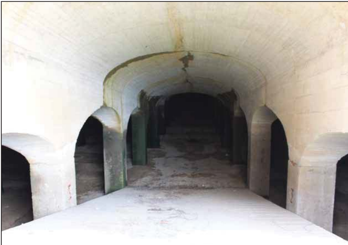
Ramp in Filter Bed 11. 2015.
