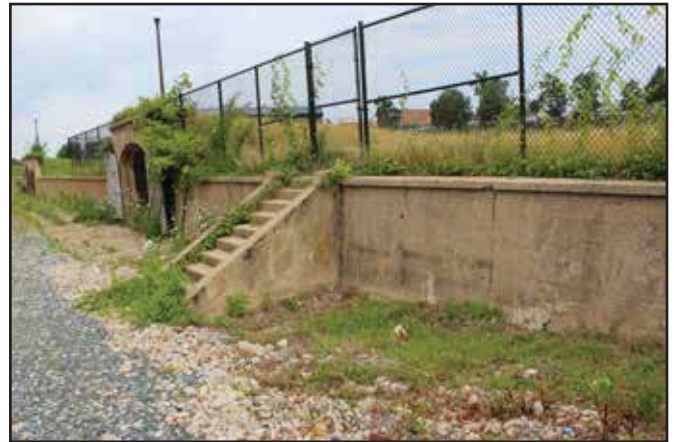
North wall at Service Court 2, at Filter Bed 14. 2015.
