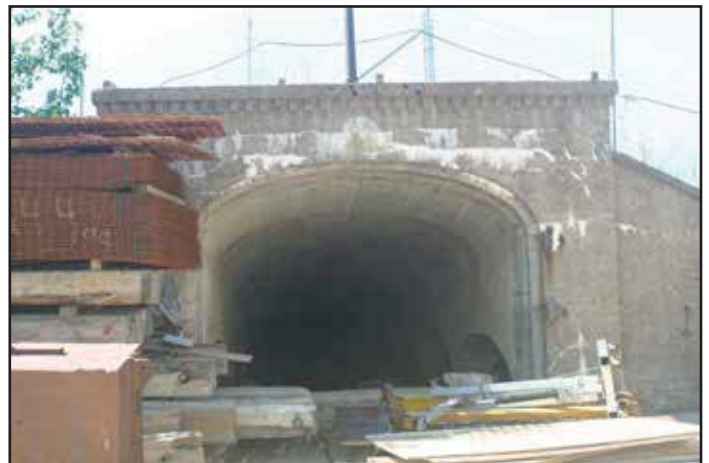
Filter Bed Portal 29. 2015.
