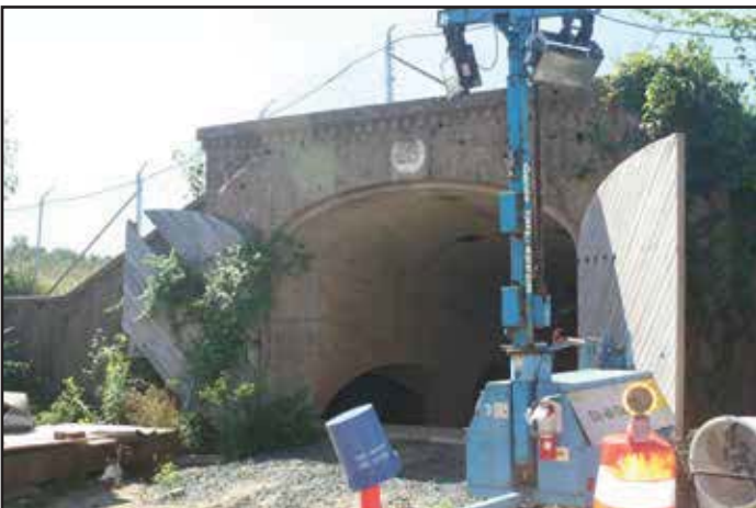
Filter Bed Portal 28. 2015.
