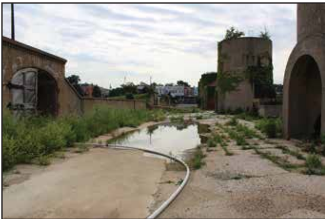
Detail of paving at Service Court 3, looking east from Sand Bin 14. 2015.
