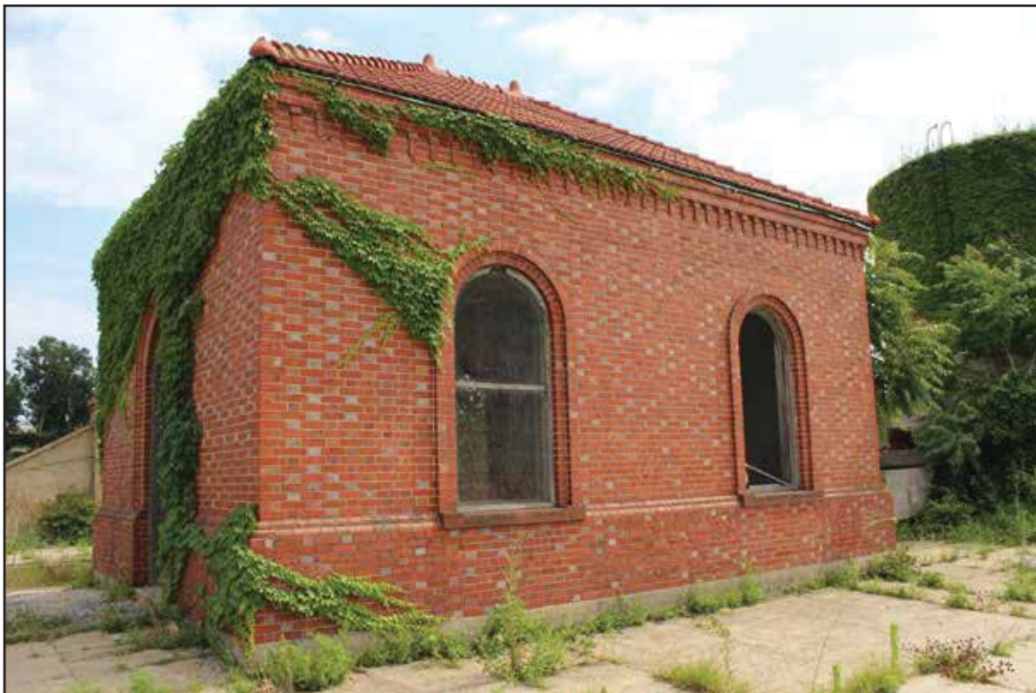
Regulator House 5, looking northeast. 2015.
