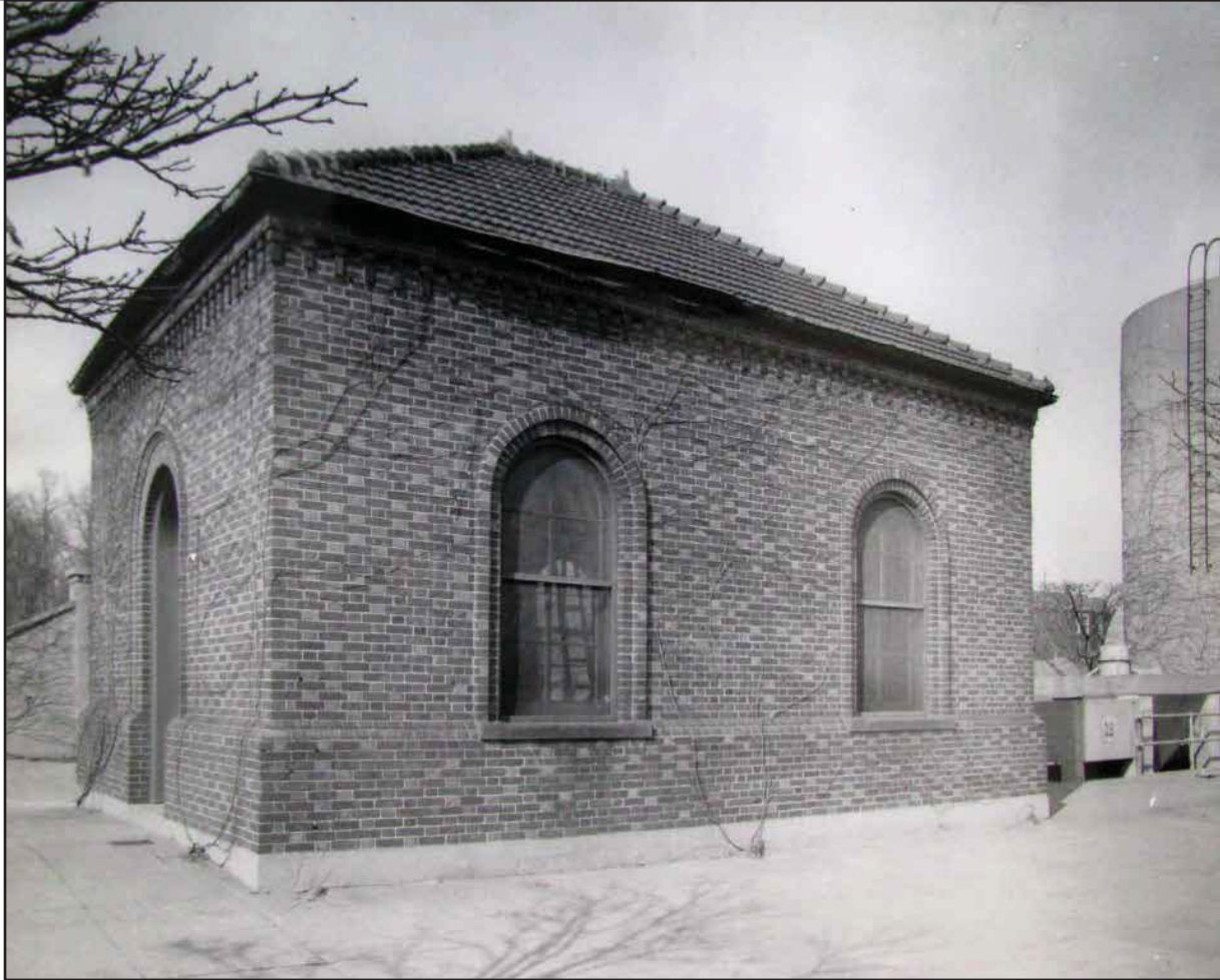
Regulator House 5, looking northeast. Circa 1944. Courtesy of the Washington Aqueduct Archives.
