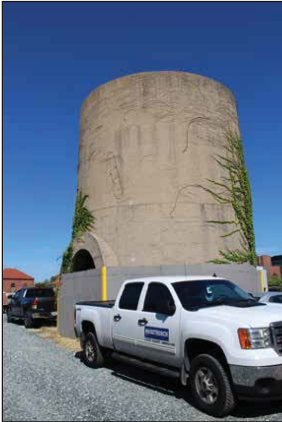
Sand bin 20, looking northwest. 2015.
