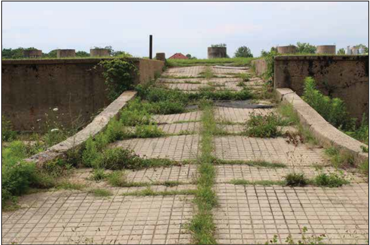
Ramp leading from Service Court 2 to top of Filter Bed 18. 2015.
