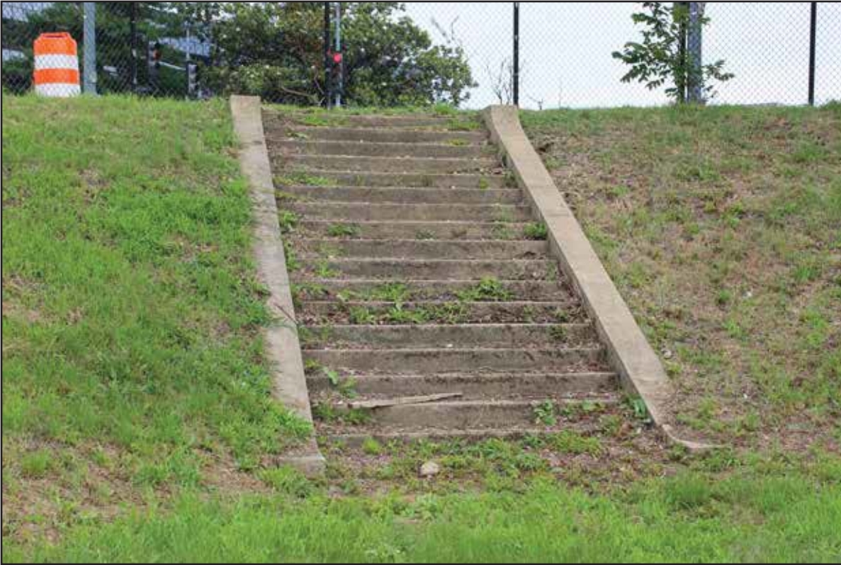
Stairs at northwest corner, looking northwest. 2015.
