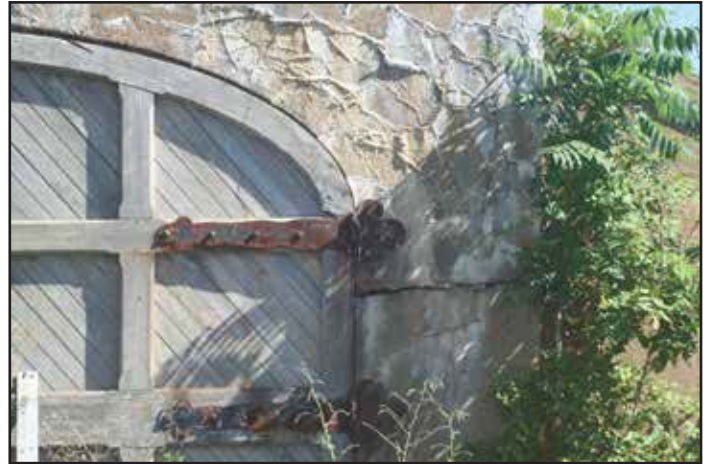
Wood door and hardware at Filter Bed Portal 24. 2015.
