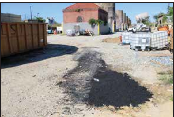
Detail of paving at Service Court 3, looking southwest from Sand Bin 27. 2015.
