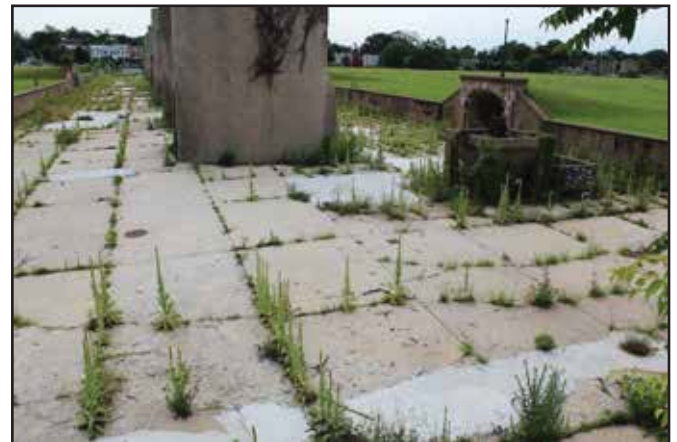
Detail of paving at Service Court 2, looking southeast from First Street. 2015.
