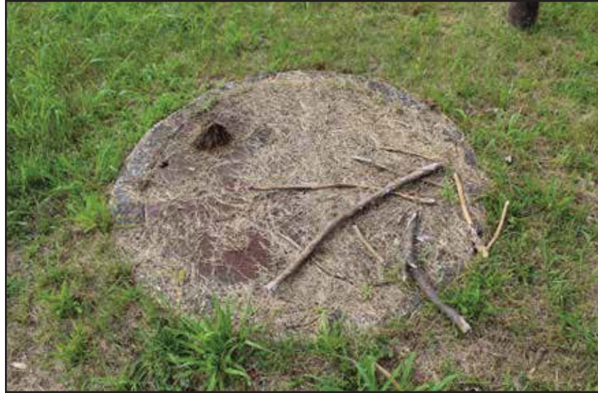
Manhole cover at southwest corner of filter bed 10. 2015.
