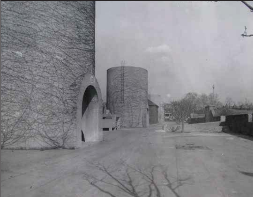
Service Court 2 from about center, looking east. March 25, 1944. Courtesy of the Archives of Washington Aqueduct
