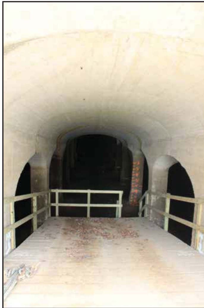
Ramp in Filter Bed 14. 2015.
